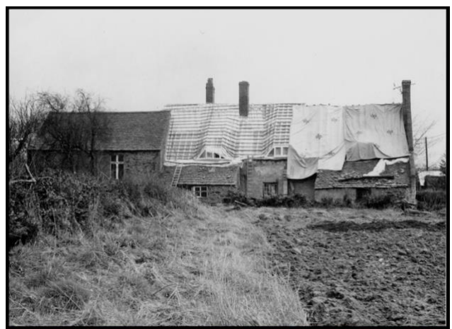
The rethatching of Canon Godfrey's cottage behind the Chapel
