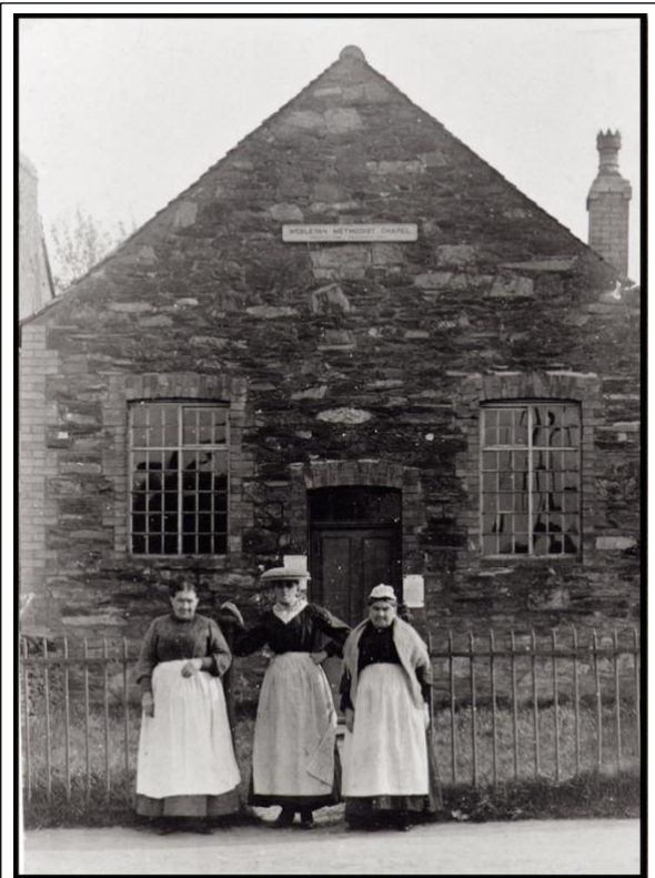
The chapel from the road showing the cast iron sign in the gable.
